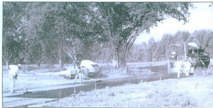
Crews pave one of the cemetery's roads.
