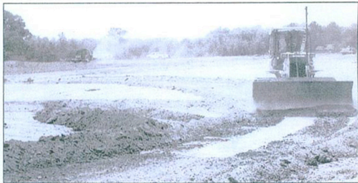
A Komatsu dozer grades the road to the maintenance area.
